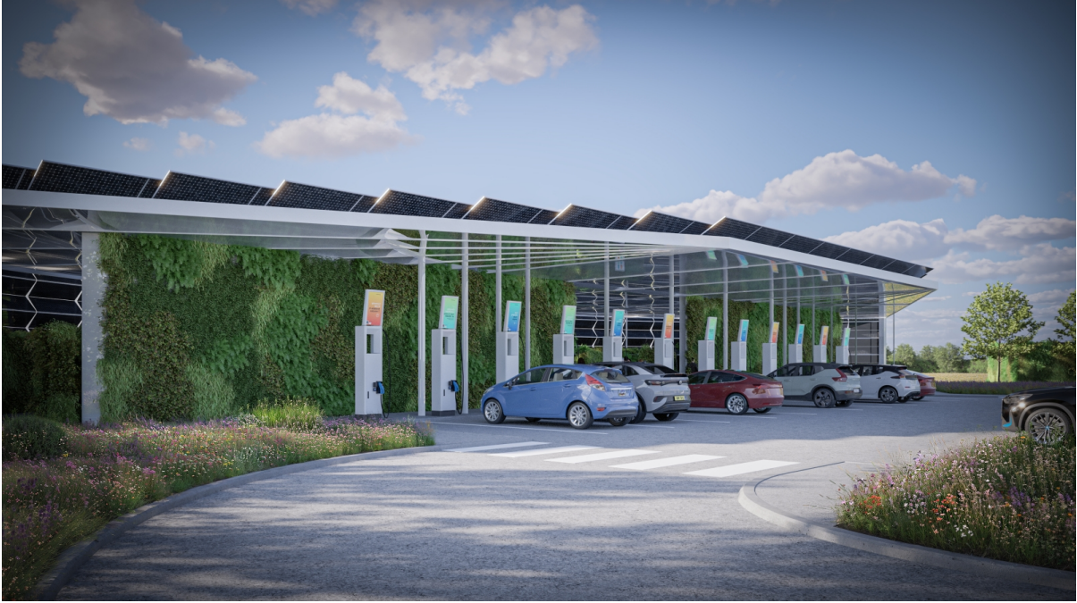
Lightstate's ultra-fast EV charging hub in the UK. Source: Lightstate Ltd.
